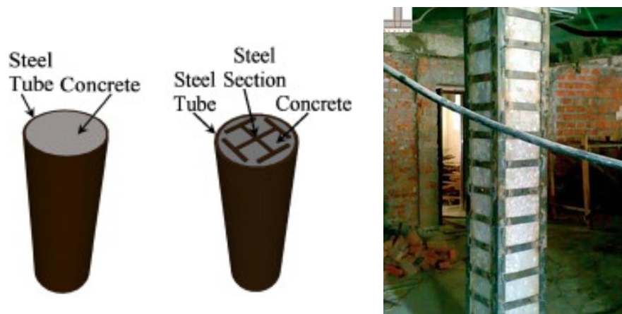
Figure 4. Steel jacketing [5, 7].
