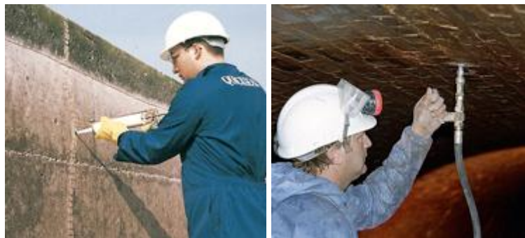
Fig 2. Resin injection on RC members/ structures [4].
